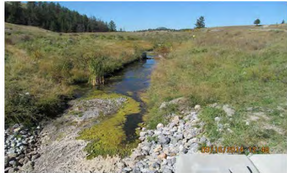
PANEL 2. UPSTREAM VIEW OF JACKO LAKE DAM AND SPILLWAY SEPTEMBER 16, 2014.
