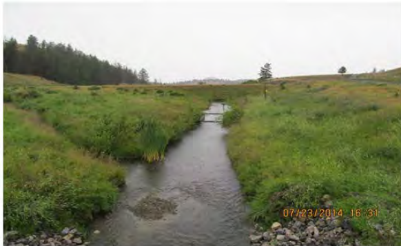
PANEL 1. UPSTREAM VIEW OF JACKO LAKE DAM AND SPILLWAY, JULY 23, 2014.
