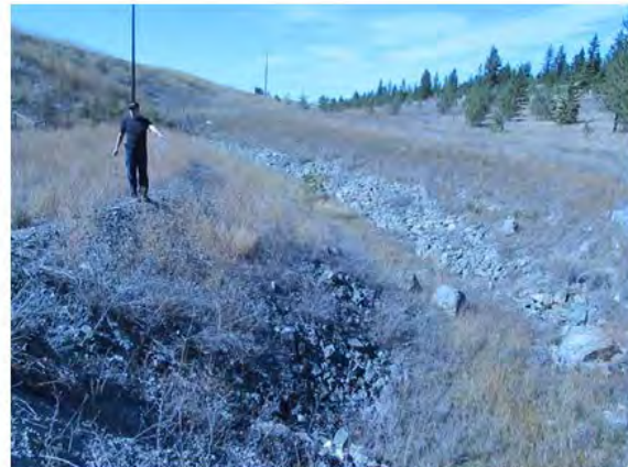
PANEL 2. VIEW NORTH OF DITCH PARALLEL TO HIGHWAY 5 ON NORTH SIDE OF HISTORICAL AFTON MINE HAUL ROAD. SEPTEMBER 15, 2014.
