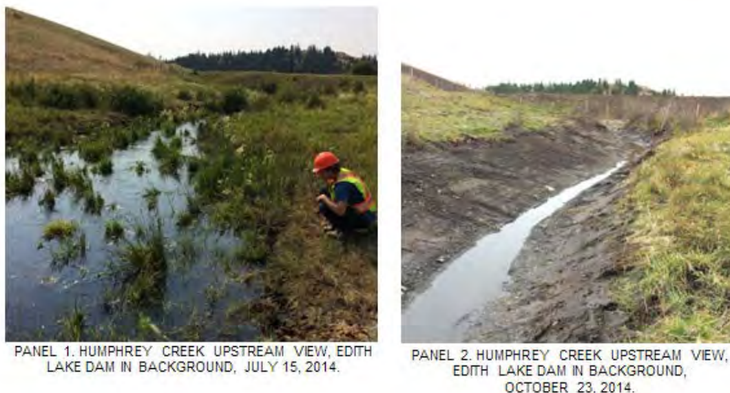
Figure 3.3-13 Upper Humphrey Creek
