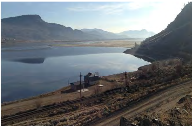
PANEL 1. VIEW EAST OF NEW AFTON WATER INTAKE SITE ON KAMLOOPS LAKE FROM ACCESS ROAD, MARCH 26, 2013.
