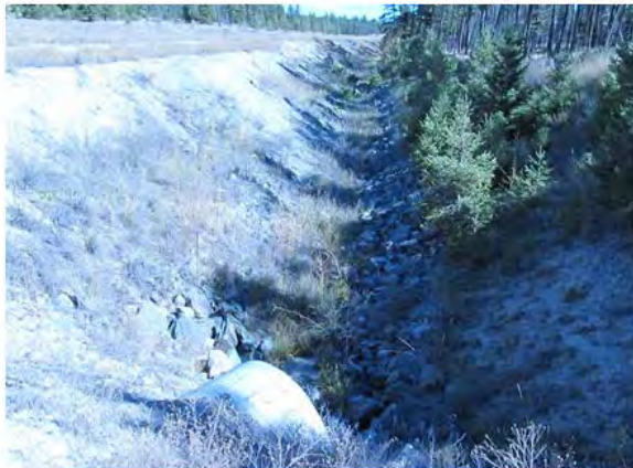
PANEL 1. VIEW EAST FROM SOUTH SIDE OF AFTON MINE HAUL ROAD SHOWING DRAINAGE DITCH AT MAPPED LOCATION OF ALKALI CREEK UNNAMED TRIBUTARY. SEPTEMBER 15, 2014.
