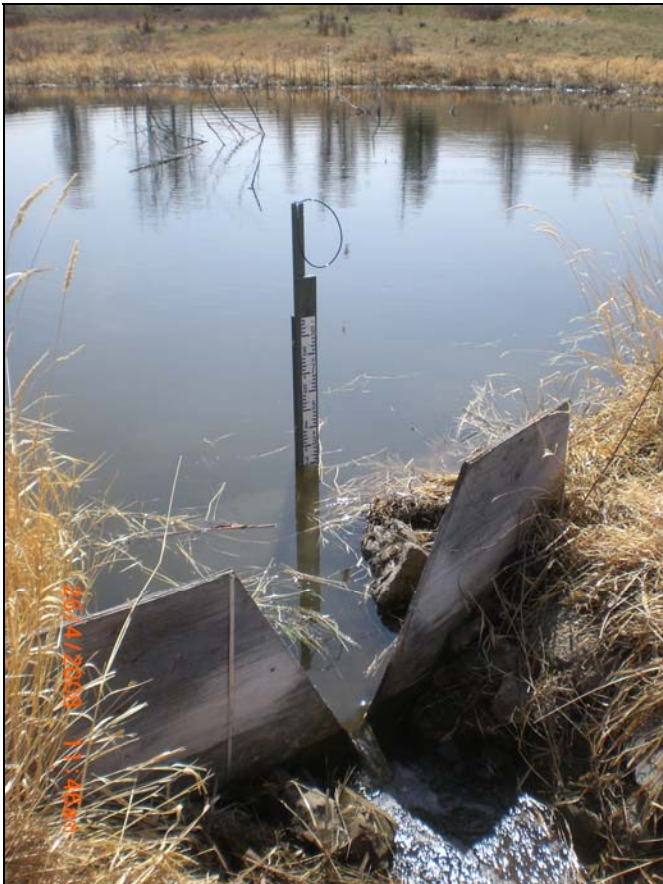
PHOTO A10 – TSFINF V-Notch Weir Control (2008)
